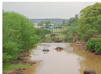
Rainwater Harvesting implementation through Borewell at Kadus
