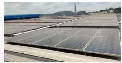
Roof Top Solar
