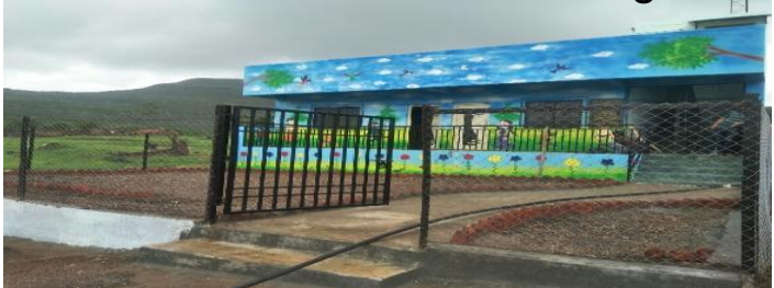
Construction of School building
